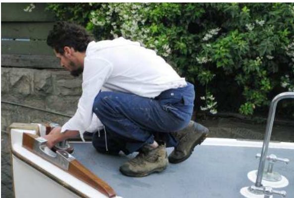
Figure 3 – Cyril Inspecting Work on MB168
