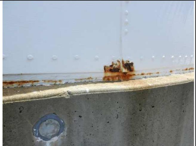
**Step 7** – The window may need to be removed and badly corroded plate underneath replaced along with the window sill. Otherwise treat overlapped areas using the same technique as steps 1 & 2 above.
